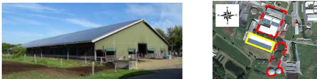
Figure 1: Left: Investigated barn. Right: Overview of the barn and its surroundings. The barn is outlined yellow; potential external pollutant sources are outlined red.
